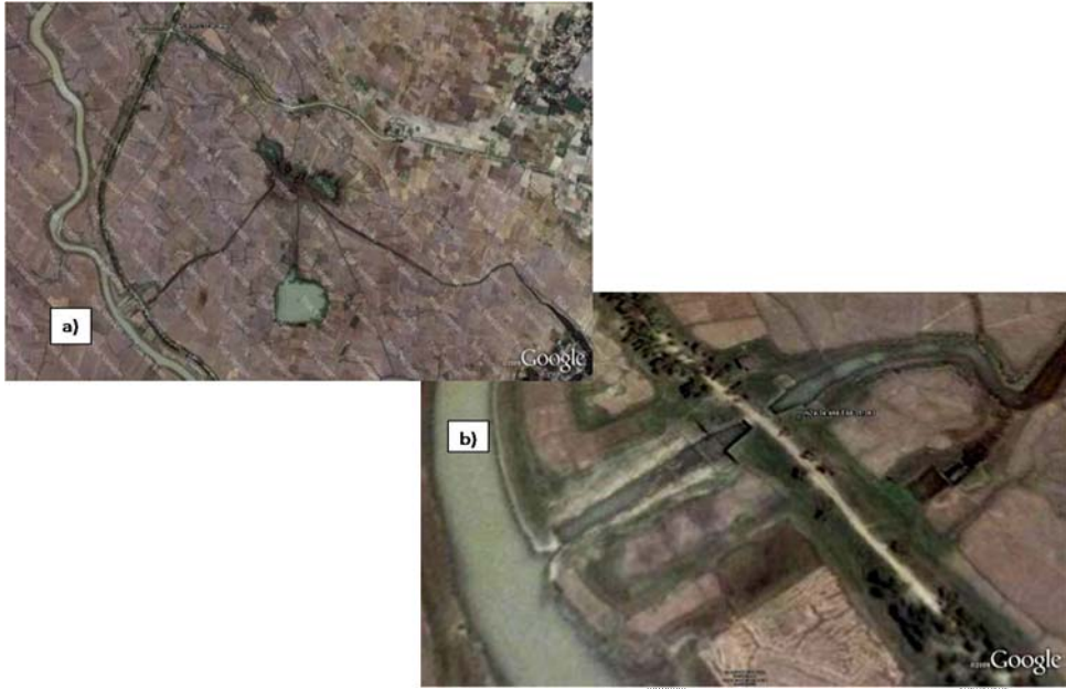
Figure 9: Beel Mail a) refuge areas remaining in the beel during dry season, b) sluice gate (image © 2009 Digital Globe, © 2009 Google)
